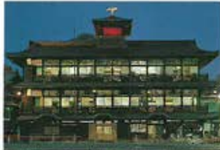
Night view of the building of Dogo Hot Spring
