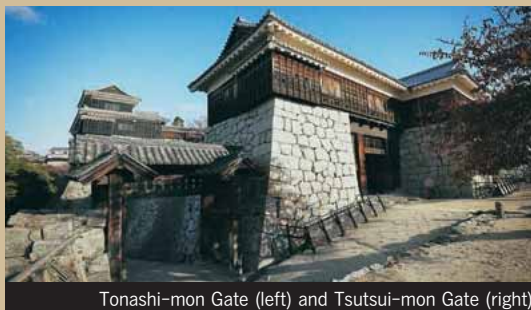
Tonashi-mon Gate (left) and Tsutsui-mon Gate (right)
