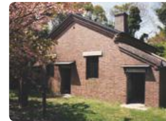
■ Remains of Power Plant
